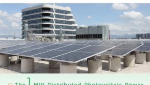
O The MW Distributed Photovoltaic Power Generation Project in Shanghai C&D Center, with an expected average annual power generation of 1, 1 million kWh
