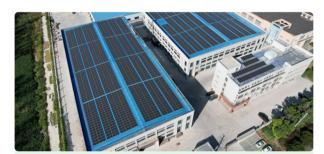
The 1.8 MW Distributed Photovoltaic Power Generation Project in Jiangsu Junda, with an expected average annual power generation of 1.98 million kWh
